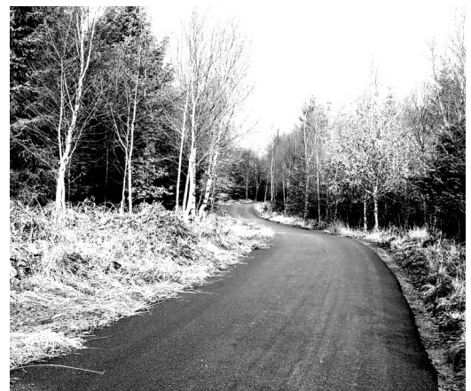
Above: Tarred Surface at South End of the Gort Daraich
